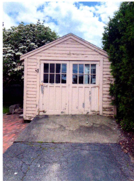
GARAGE EXIST FRONT
