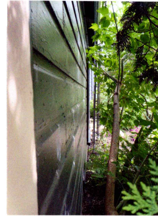
GARAGE EXIST RIGHT SIDE
